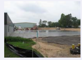
Foundation was laid July 2010.
