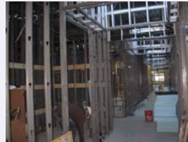
Inside office walls were placed October 2010.
