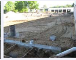
Footings for the addition were laid down July 2010.
