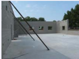
Inside Walls were erected August 2010.
